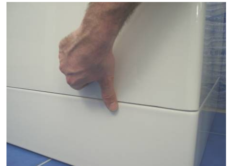
6/ Refit panels and ensure a good aesthetic result is achieved .
