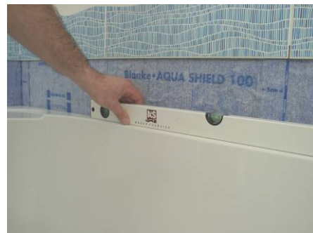
7/ Re-check the level of the bath along both the width and length using a spirit level, Adjust feet if necessary to ensure bath is level and stable.
