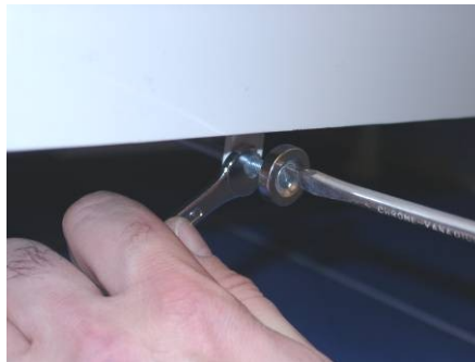
5/ Adjust threaded magnets to adjust panels in/out to suit.
