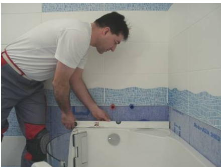
7/ Re-check the level of the bath along both the width and length using a spirit level, Adjust feet if necessary to ensure bath is level and stable.
