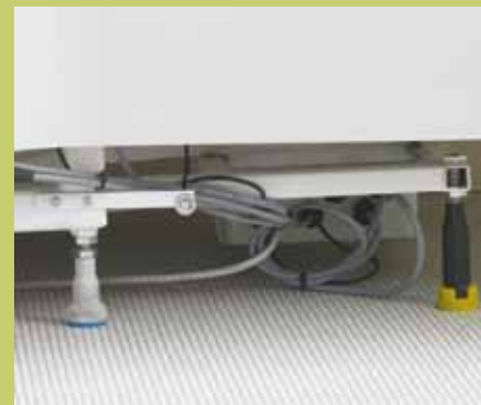
Electronic box sits neatly into metal brackets under bath for access. Magnetic plinth brackets
